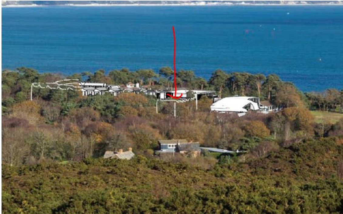
Figure 6.7 – view 5b wireline from Appendix 6.5 in the submitted EIA (CD1.059) – the two storey villa shown in outline (red arrow) is not appearing in photomontage
