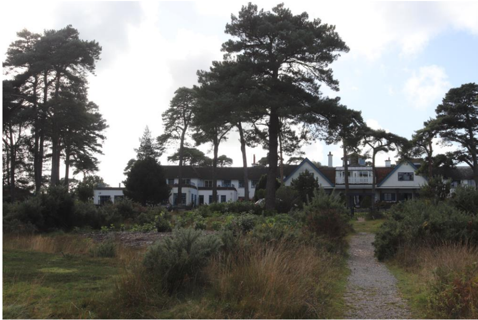
Figure 4.3: View of eastern elevation of existing hotel – illustrating character of existing building
